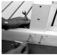
Place Chaise Body Assembly face down on a clean flat surface. Place Rear Legs inside Chaise Body Assembly, while aligning predrilled holes. Rear Legs have to holes extra for Wheels. Attach using (2) 2-3/4" connector bolts, flat & lock washers and nuts (Left Picture). Repeat process on other side and for Front Legs (Right Picture).
