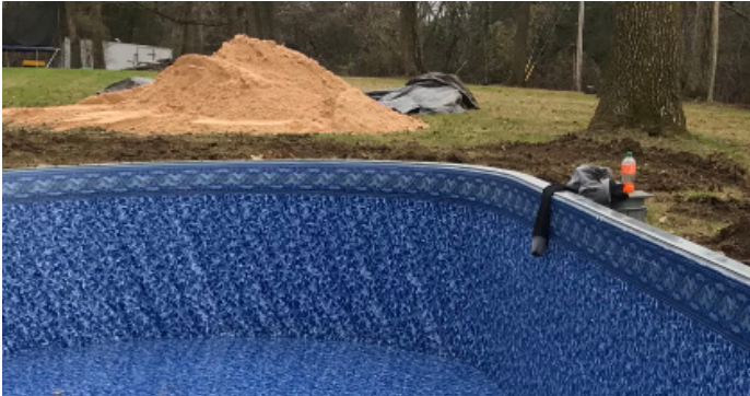
This is left over pool sand on the job site. It is more cost saving to order more sand and have a little left over than to order and pay another delivery charge if you don't have enough.
