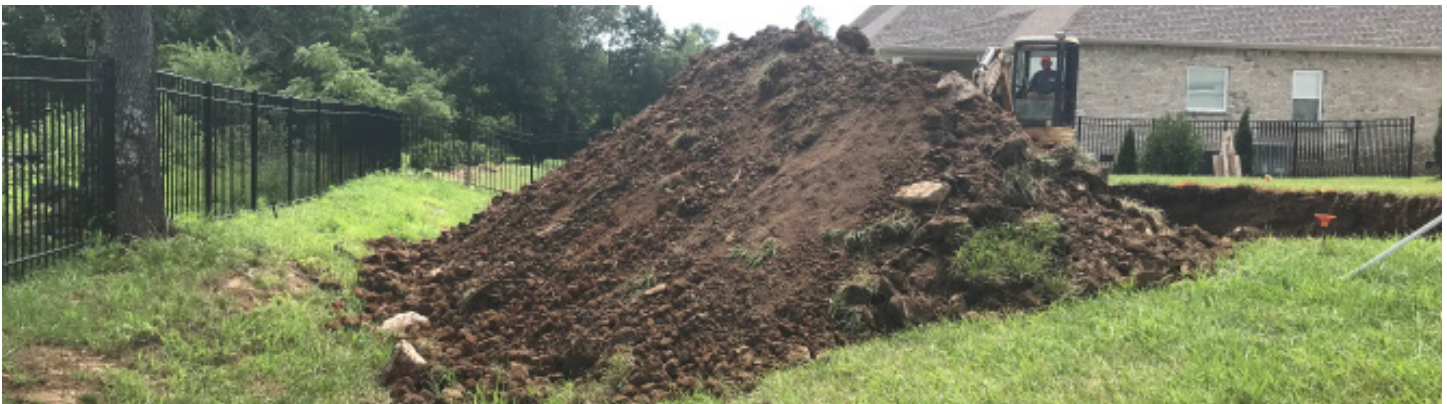
This picture shows where a homeowner asked us to move the dirt to the end of his property. This can be done by paying the excavator directly after the pool is installed. A local excavation Company can be found to move dirt and grade your yard after the build for an affordable rate.
