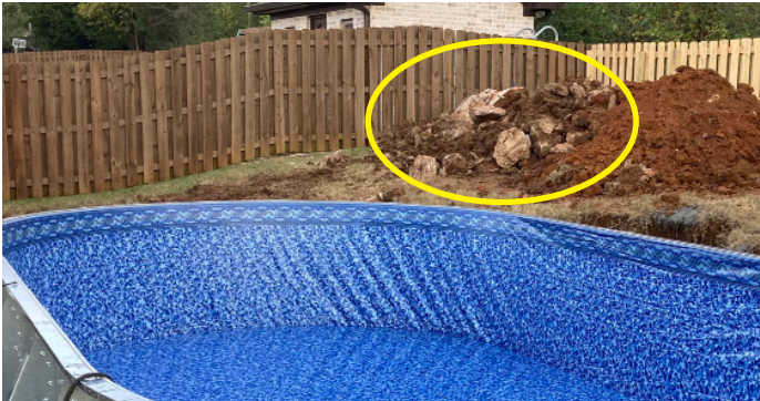
Some jobs have a little rock in the ground when we dig, so be aware that your yard could have the same. It is important for the bottom of the pool base around the outside to have dirt pushed up around it to help contain the sand.
