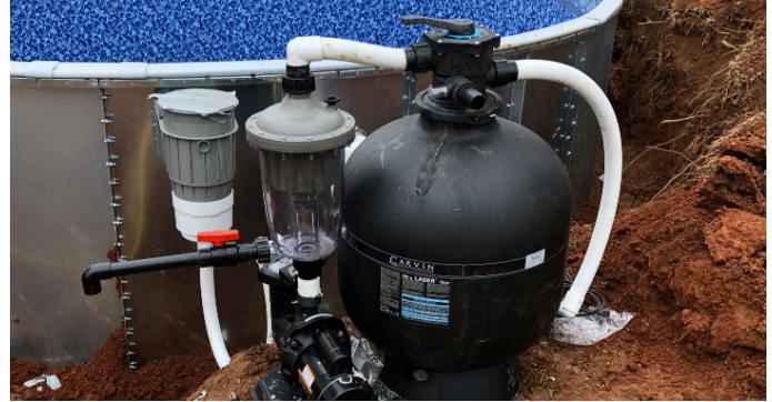
This is a picture of your pump and filter. Notice the dirt ground after digging out the pool. This is very common, and most homeowners plant seed and straw to grow back the grass after installation, or you can use decorative gravel.
