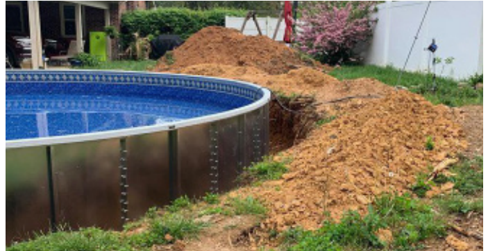
This pool had a very small slope, but you can see how much dirt is left behind. Additional excavation, grading and dirt work may be available by bid only, made prior to install date, and paid directly to the excavator.
